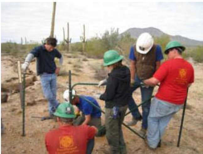
Roy and the SCC crew put up fencing at the end of Smith Road (8022).
