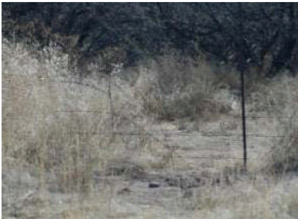
Photo F (Damaged Border Fence)
